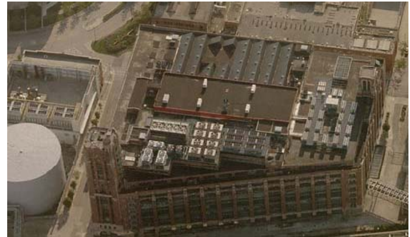
Lakeside Technology Center, Chicago 1 100 000 fs, 100 MVA
